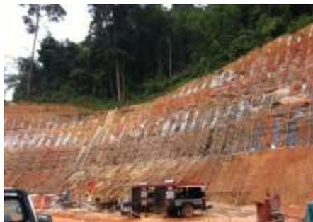
Soil nail is commonly used in Malaysian slopes both as a stabilization measure for distressed slopes and for very steep cut slopes. The popularity of soil nail slope is due to its technical suitability as an effective slope stabilization method, ease of construction and is relatively maintenance free. As such, soil nail slope of up to more than 25m high is increasingly being used for Malaysian slopes.
